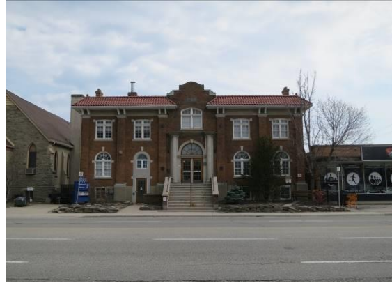
Figure 12: Clark Memorial Hall, 161 Lakeshore Road West
