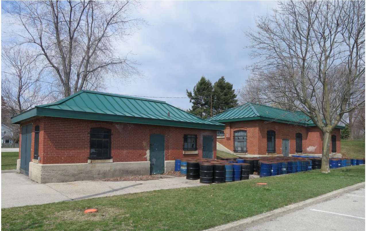
Figure 39: Two of the former waterworks buildings located in J.C. Saddington Park. Adaptive re-use of these buildings is recommended. Credit: GRA.
