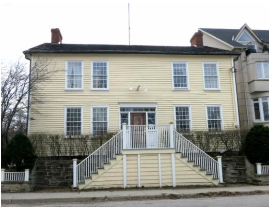
Figure 9: The former Wilcox Inn, 32 Front Street.
