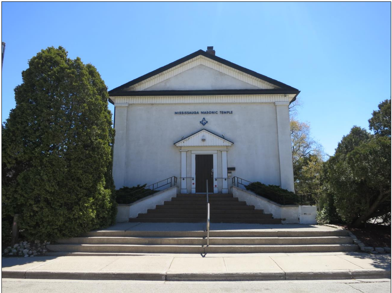
Figure 8: Mississauga Masonic Temple, built in 1926, incorporates within its walls the Wesleyan Methodist Church of 1849, the first church in Port Credit. Credit: GRA.
