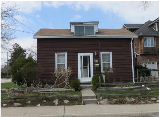
Figure 13: Vernacular dwelling, 48 Lake Street
