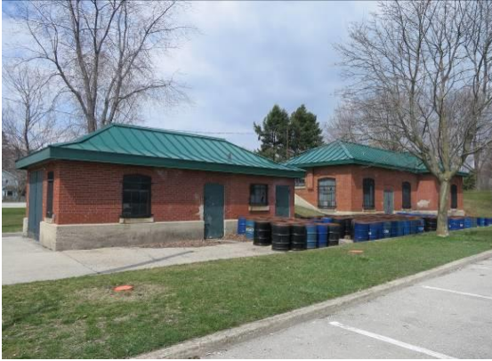
Figure 11: Village waterworks buildings in J.C. Saddington Park
