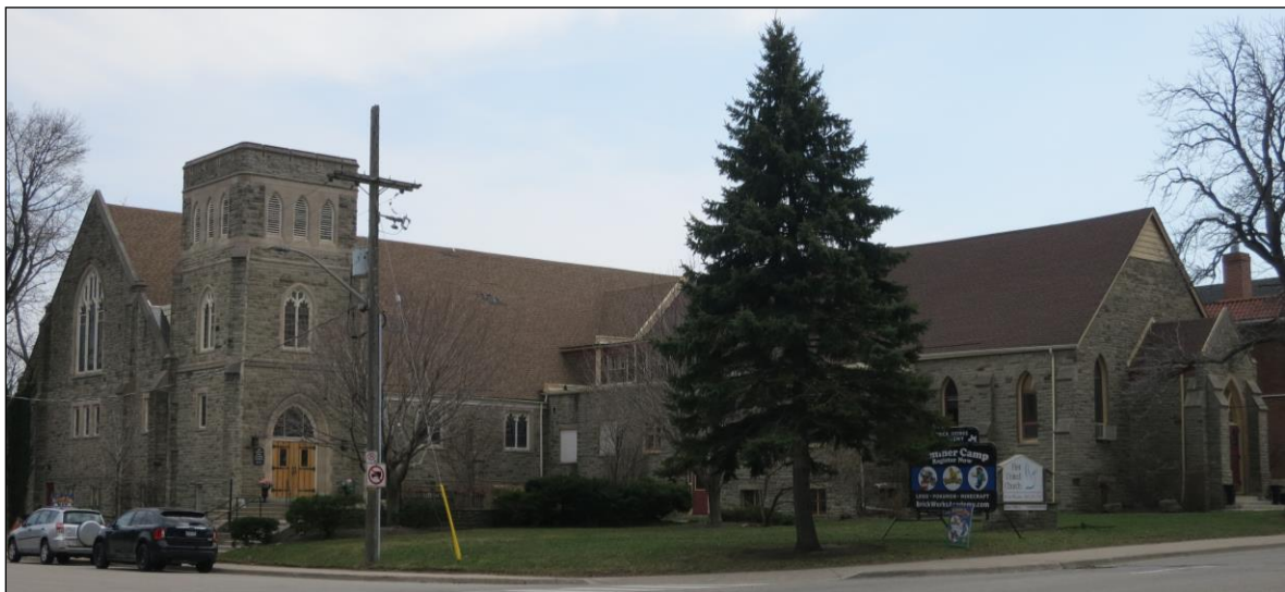
Figure 7: The private open space of institutional buildings is an important landscape feature along Lakeshore Road West. Credit: GRA.
