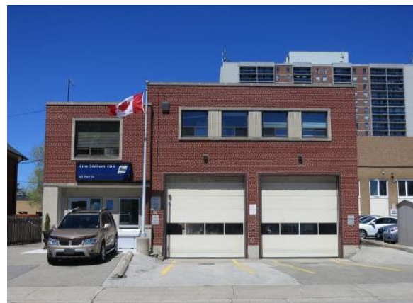
Figure 10: Fire hall, 62 Port Street
