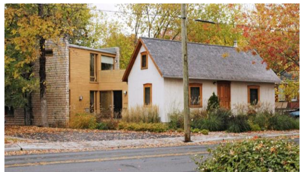
Figure 26: An example of a suitable contemporary addition with the preferred materials of wood and shingle siding. The scale is preferred, and is the differentiation between old and new construction. Credit: Atelier Pierre Thibault / Alain Laforest, photographer.
