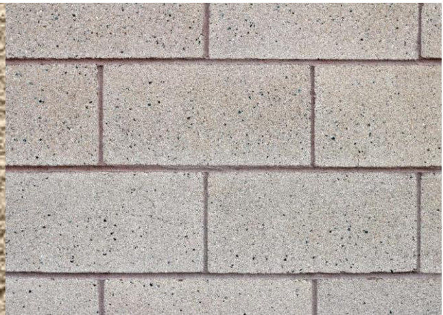
× Discouraged: exposed concrete block
