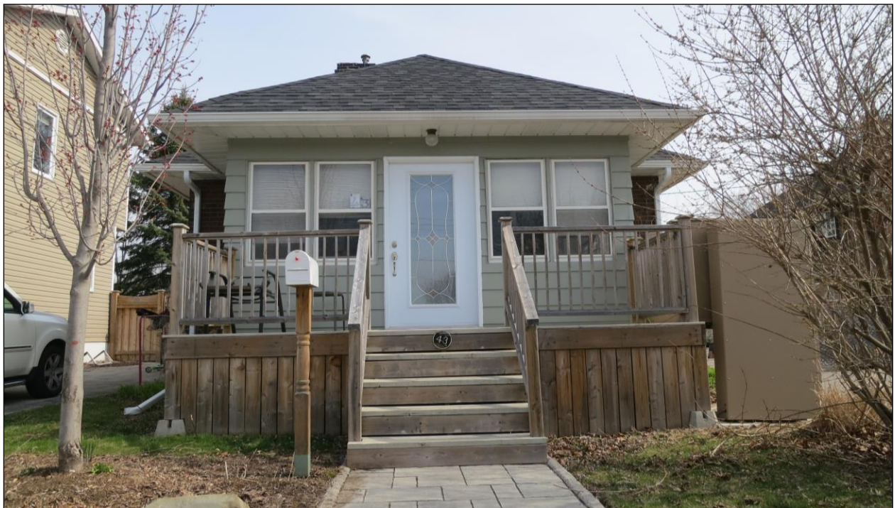
Figure 46: An example of an acceptable exterior barrier-free lift in the District, at 43 Peter Street South. The lift is suitable because it is not directly attached the heritage building fabric.
