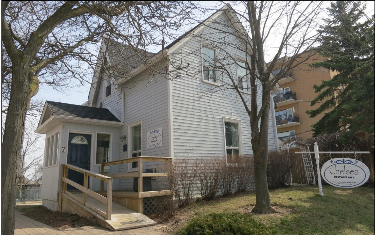
Figure 47: An example of an acceptable exterior barrier-free ramp in the District, at 7 John Street South. The ramp is suitable because it is not permanently impacting the heritage building fabric.
